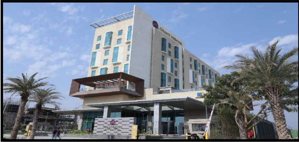
Brigade Group Hotel - 150 Rooms
